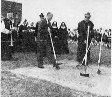
START OF A BUSY WEEKEND —Archbishop Schulte turns a shovel of dirt at the groundbreaking ceremonies at Our Lady of Grace Convent, Beech Grove, last Friday morning marking the start of construction for a $210,000 novitiate wing. At left is Beech Grove mayor Elden Geshwiler, R. Rev. Archabbot Ignatius Esser, O.S.B., convent chaplain, is at the far left. Between Mayor Geshwiler and the Archbishop are Rev. Mother Mary Robert, O.S.B., prioress; and Sister M. Cleophas, O.S.B., subprioress. The wing will provide facilities for 72 Junior Sisters during the Sister-Formation period.
