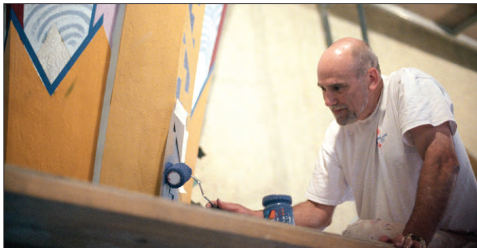
A Conrad Schmitt Studios employee from New Berlin, Wis., paints a section of the church ceiling outlined by stencils during replication work on a ceiling arch in May.
