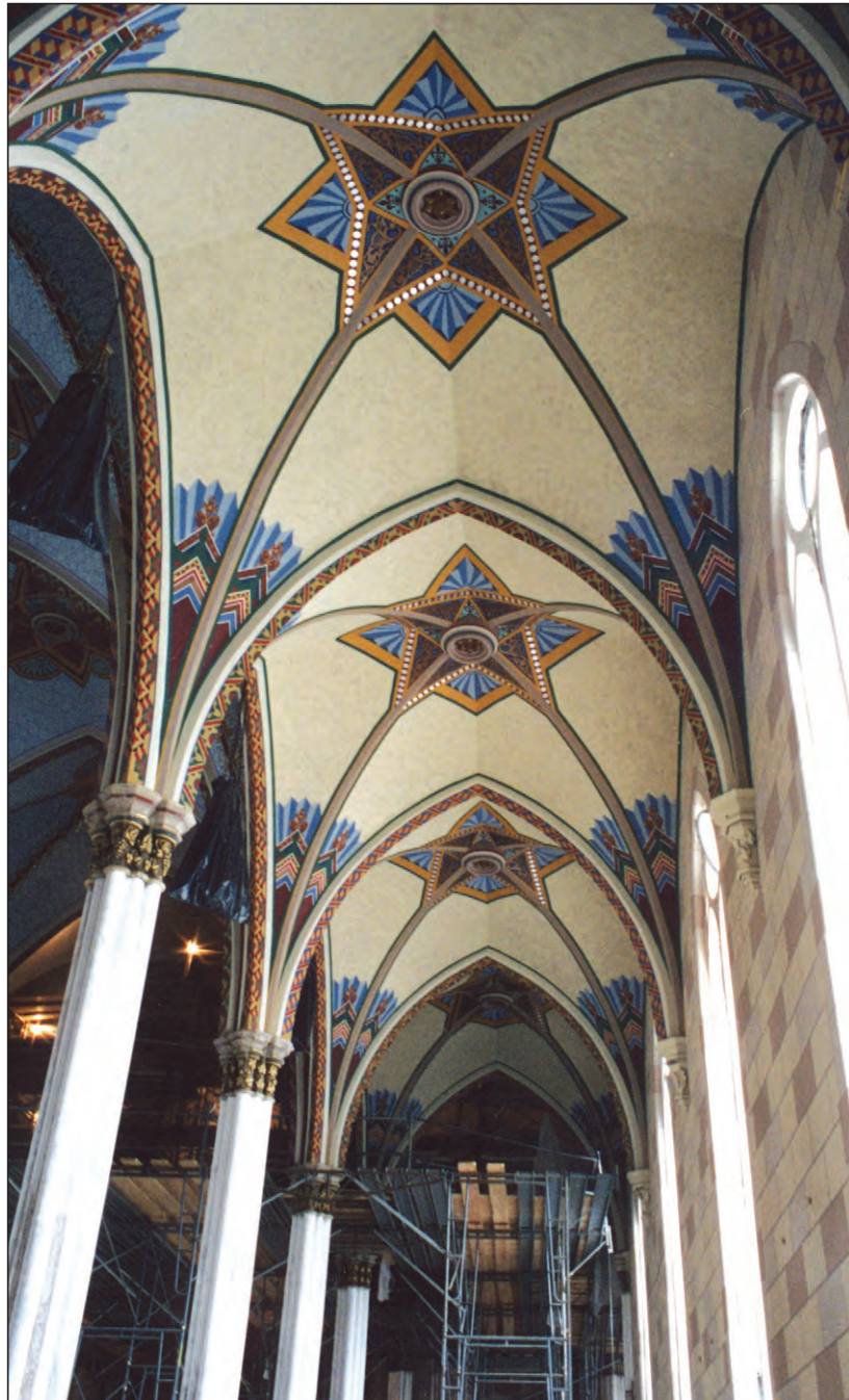
Replication of decorative painting on the ornate, arched ceiling of Sacred Heart of Jesus Church in Indianapolis was recently completed by employees of Conrad Schmitt Studios of New Berlin, Wis. The historic 121-year-old church was extensively damaged by an electrical fire on April 27, 2001.
