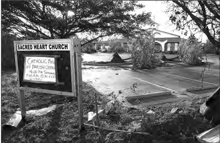
Sacred Heart Catholic Church in Punta Gorda, Fla., sits amid downed trees and building rubble and debris in the aftermath of Hurricane Charley, which made landfall in this southwest Florida city on Aug. 13. Despite extensive roof and water damage that rendered the building uninhabitable, it was reported that the sanctuary candle, indicating the presence of the Blessed Sacrament, was not extinguished and continued to burn.
