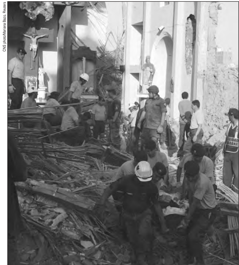
Rescue personnel work at a destroyed church in Pisco, Peru, on Aug. 16 after a major earthquake struck the evening before, killing hundreds of people, mainly south of Lima.
