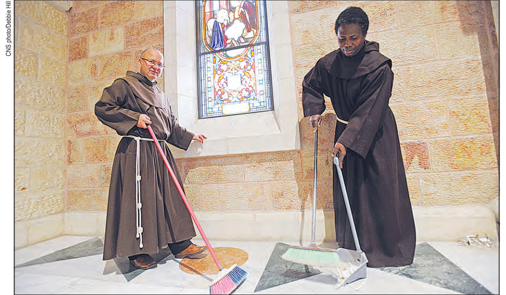
Polish Franciscan Father Jerzy Kraj and Franciscan Brother John Bomah of Ghana sweep up debris left from renovations in the Church of St. Catherine in Bethlehem, West Bank, on Nov. 26. The church, located within the Church of the Nativity complex, was undergoing some refurbishing before Christmas.
