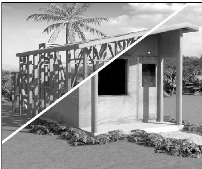
At left, a rendering showing both the frame and tented covering of the house. At right, the final version of the house with the stucco exterior in place.
