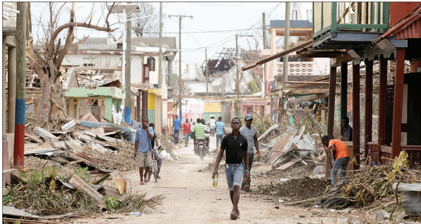
People walk past damaged buildings on Oct. 9 after Hurricane Matthew swept through Port-au-Prince, Haiti. (CNS photo/Andres Martinez Casares, Reuters)
